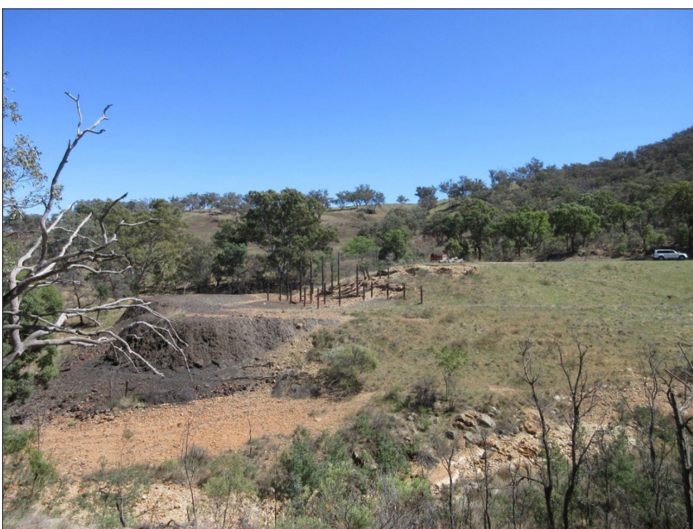
FIGURE 4: Metalliferous slag heap generated from mineral processing operations at the historic Commonwealth Mine.
